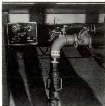
Bottom load hook-up for avgas.
